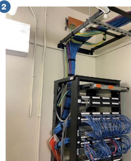
Photos, clockwise from top left: 1. A single wall-mount cabinet is installed in the secured dedicated space. 2. Proper vertical and overhead cable management, and grounding systems are used in the space. 3. A few non-IT items are stored in the space. 4. Horizontal cable supports are lacking at the cabinet and abandoned cables have not been removed from the rack.
