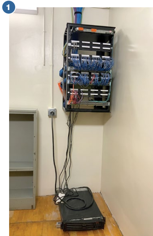
Photos, clockwise from top left: 1. A single wall-mount cabinet is installed in the secured dedicated space. 2. Proper vertical and overhead cable management, and grounding systems are used in the space. 3. A few non-IT items are stored in the space. 4. Horizontal cable supports are lacking at the cabinet and abandoned cables have not been removed from the rack.
